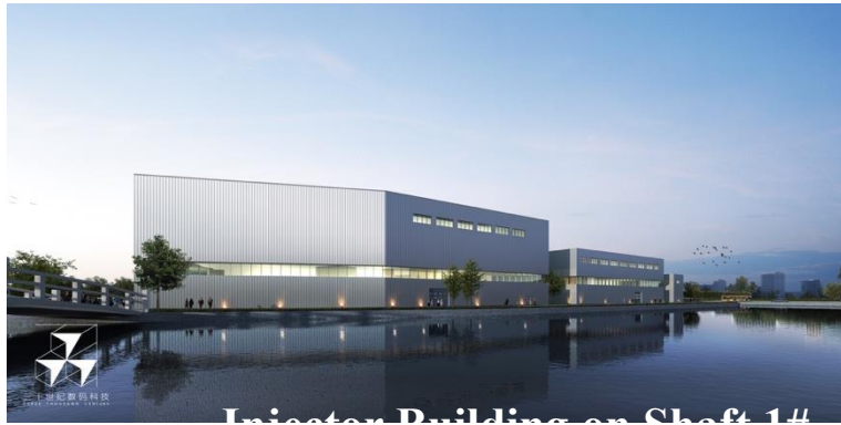
Injector Building on Shaft 1#
