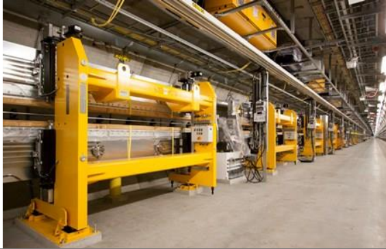
Typical, 1 FEL / 4.5m tunnel, EXFEL
